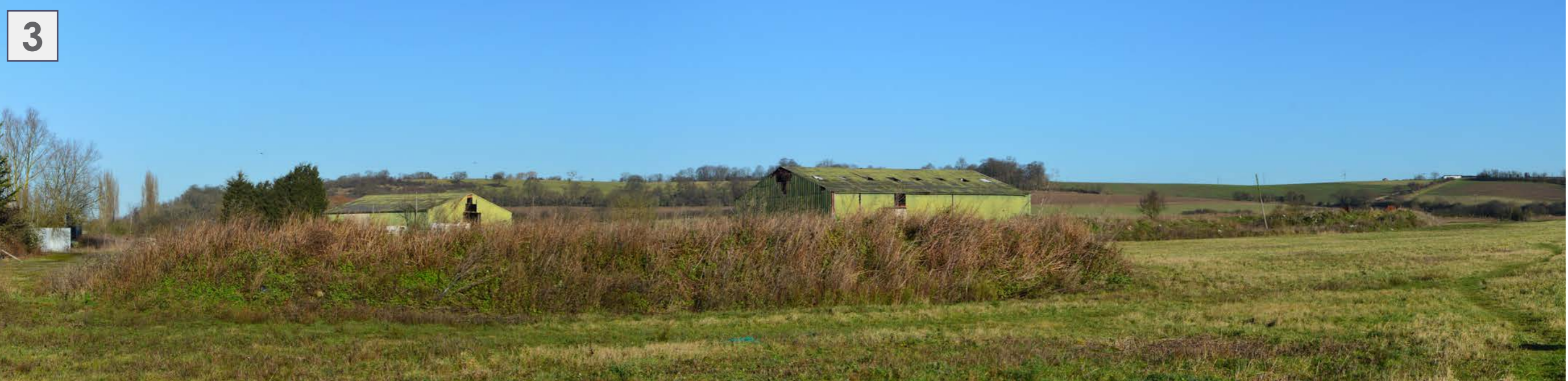
VIEW OF EXISTING STRUCTURES IN WEST OF SITE (TO BE DEMOLISHED)
