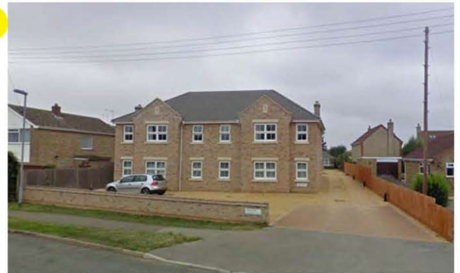
Florence House, Main Street
