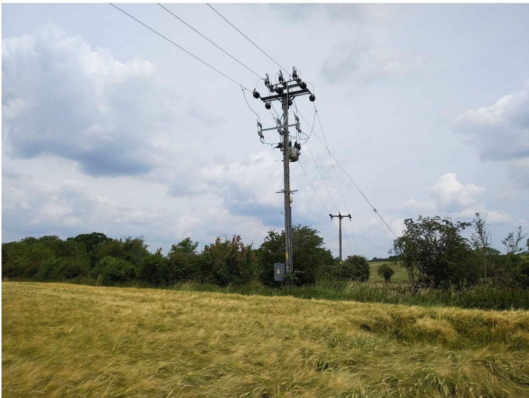
Plate 12 – Pole mounted electrical equipment on the eastern site boundary
