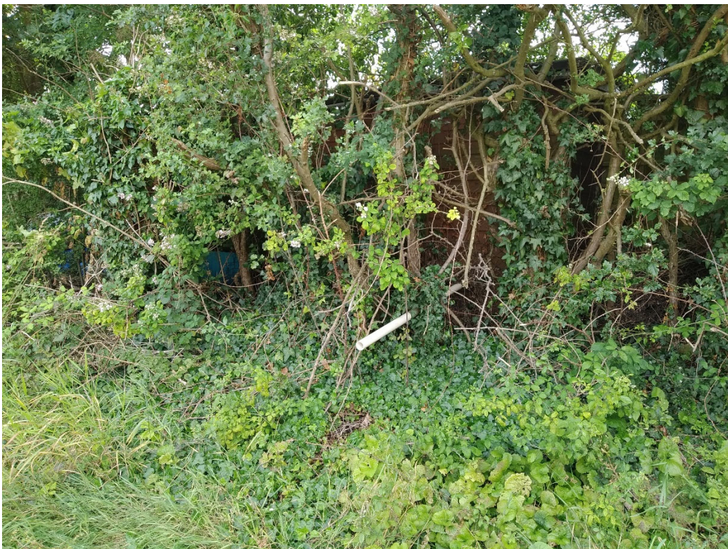
Plate 8 – Pipe from shed in the site in the south-east corner
