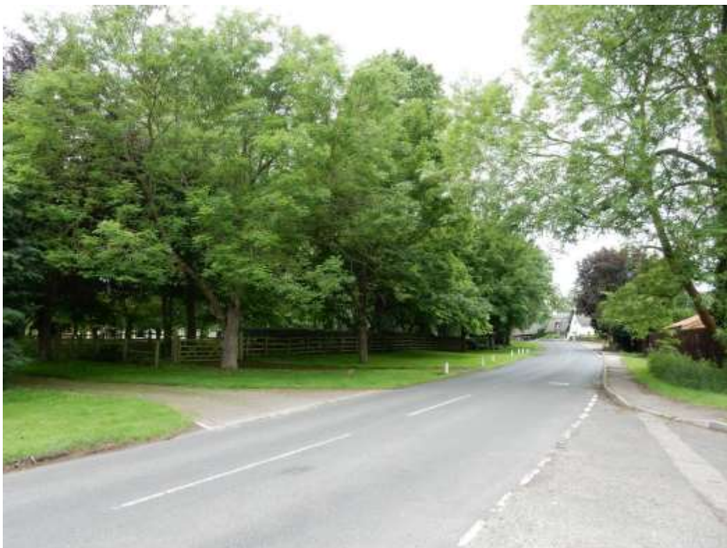
Plate 12: View north-west along Ravensden Road, with Abbey Farmhouse behind the fence and trees on the left and Nos.27-35 terminating the view ahead
