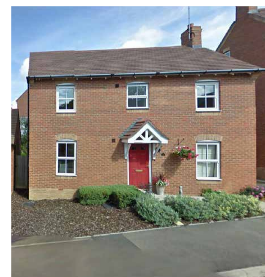
Eastfields - Modern detached dwelling built in a Victorian style in red brick with arched brick headers and white fenestration.
