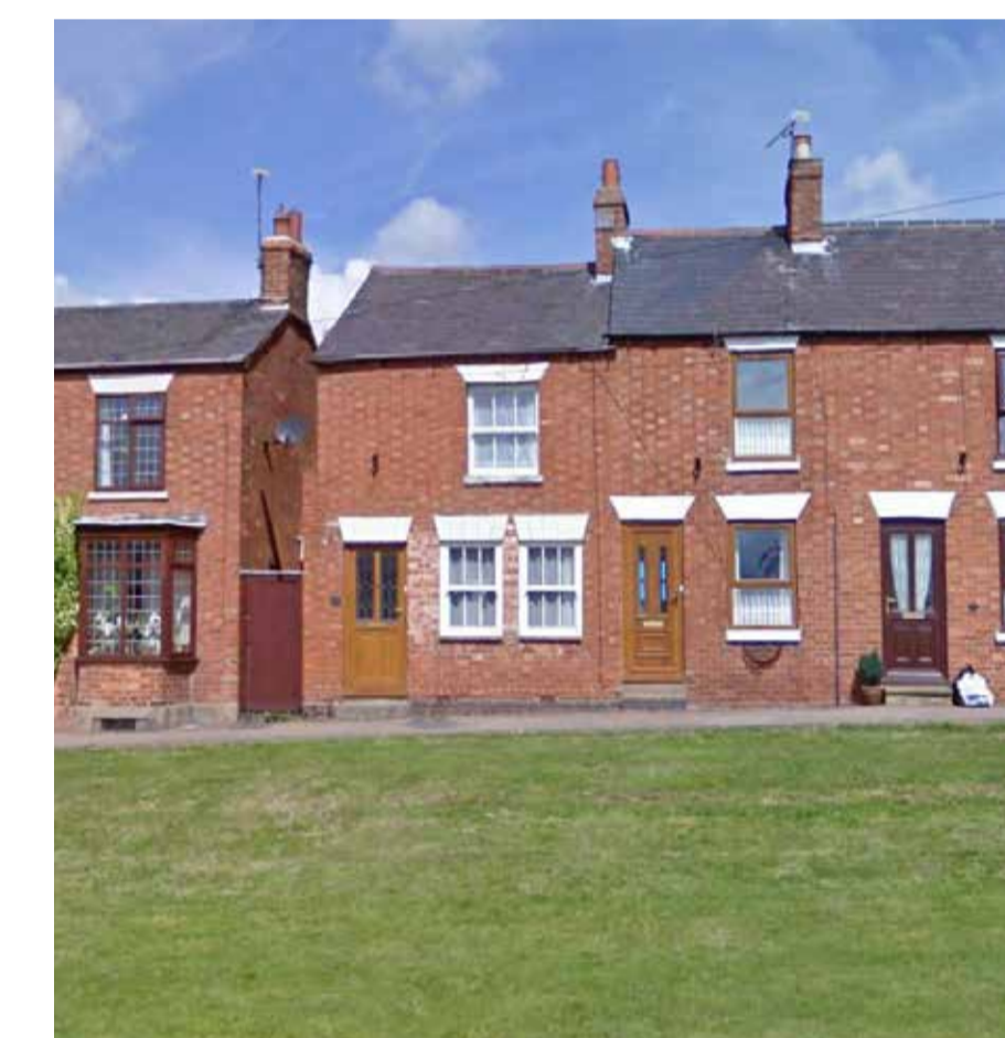
The Green - Short Victorian terrace built in red brick with stone headers and a Welsh slate roof covering.
