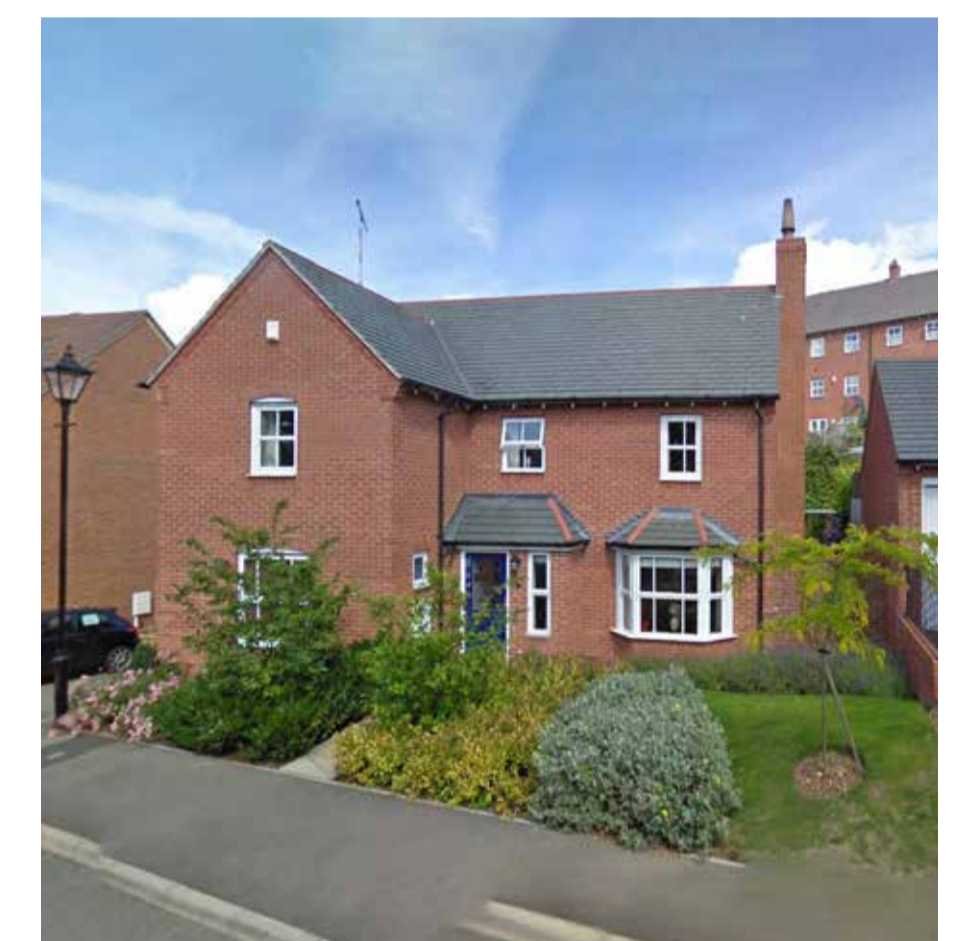
Eastfields - Modern detached dwelling built in a Victorian style in red brick with projecting gable and bay window.
