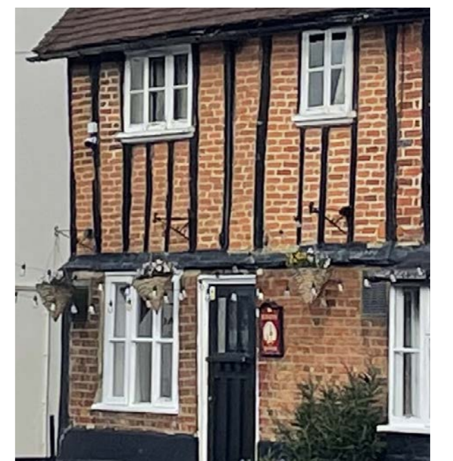
TIMBER BOARDING ON BRICK FINISH
